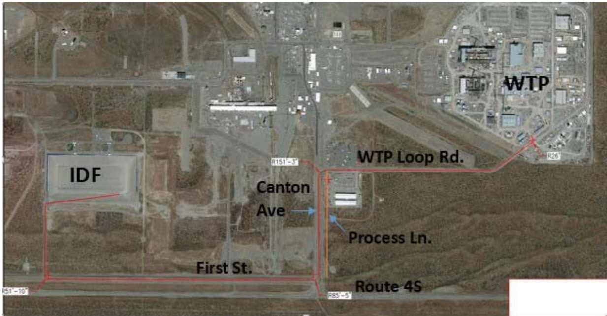
Figure 2: Roads Supporting WTP Immobilized Waste Shipments
